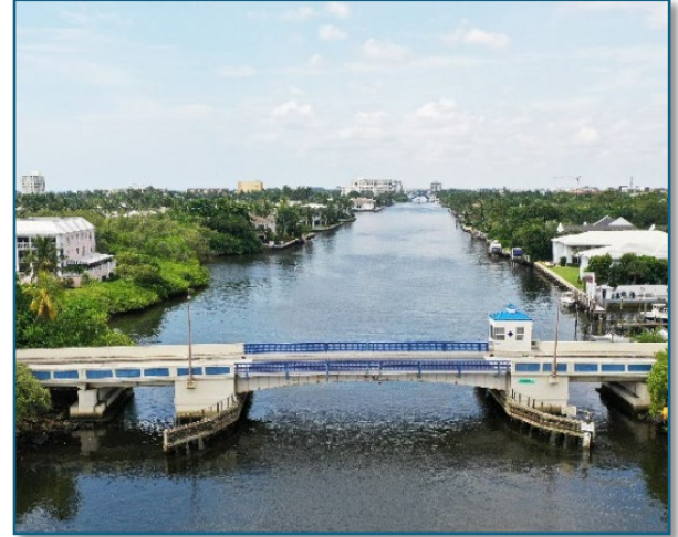
Figure 1. George Bush Boulevard Bascule Bridge
